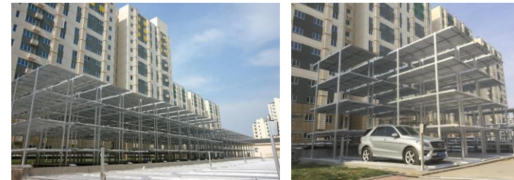
8、Residential parking garage project in BeiJing, PJS, 4/5 floor, Number of Parking Lot 115
